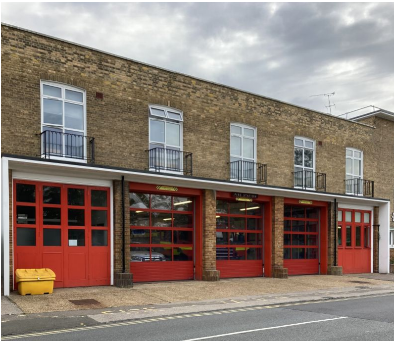
Epsom's Church Street Fire Station
