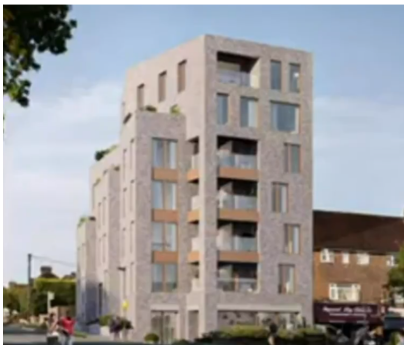
Image of original 6 storey block
