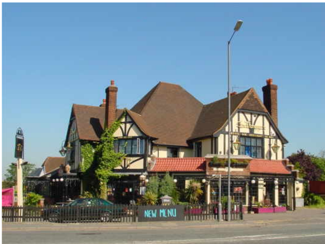
The Organ Inn before demolition. Image courtesy Peter Reed Epsom and Ewell History Explorer. Top Image: The site viewed from Ewell Bypass.
