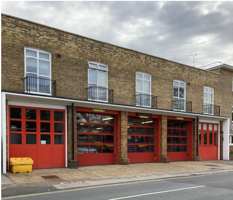
Epsom's Church Street Fire Station
