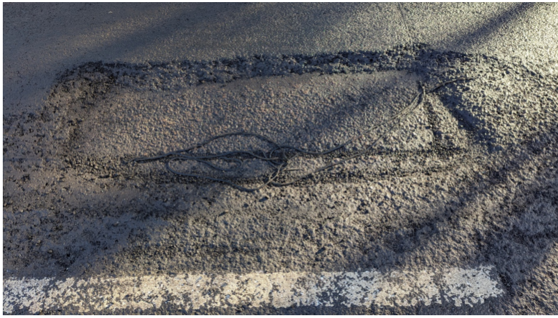
Cable exposed by pothole
