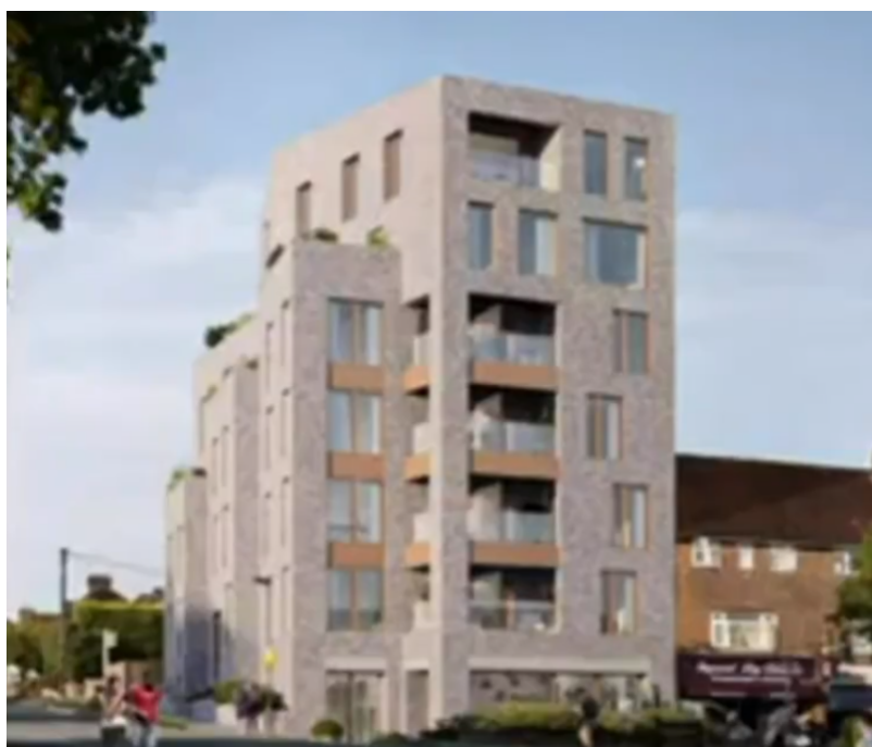
Image of original 6 storey block
