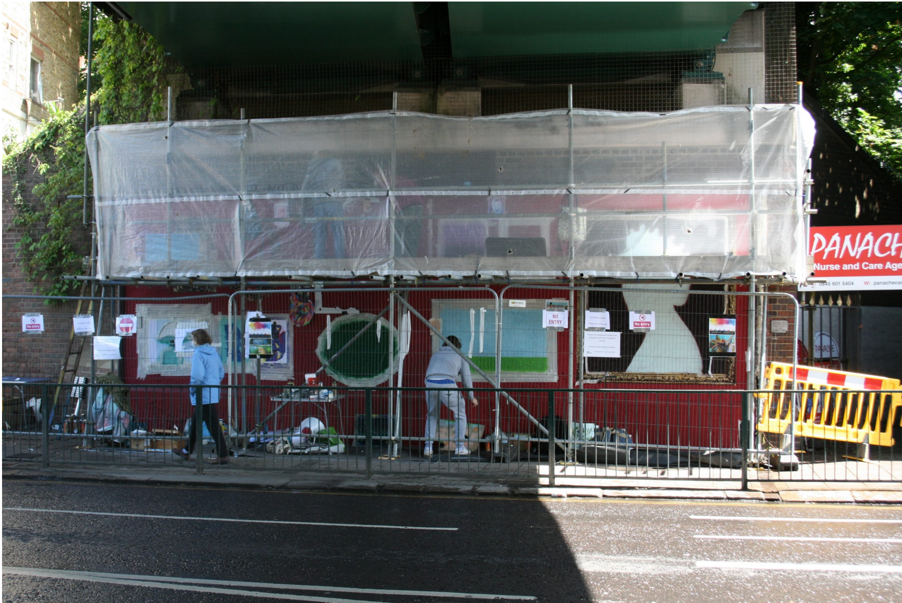
A mural being created under the East Street Bridge
