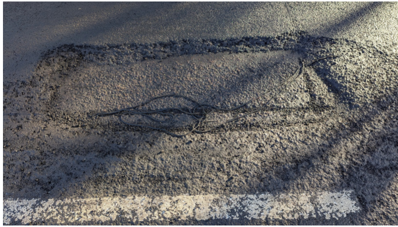
Cable exposed by pothole
