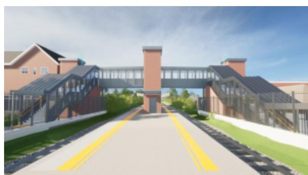
A new, covered footbridge will replace the existing structure at Stoneleigh station, providing full access via lifts or stairs to the central platform from both sides of the station. New lighting and security cameras will be installed on and around the lifts and bridge. The existing bridge structure will be removed, with the ticket office sited on the central island platform.
