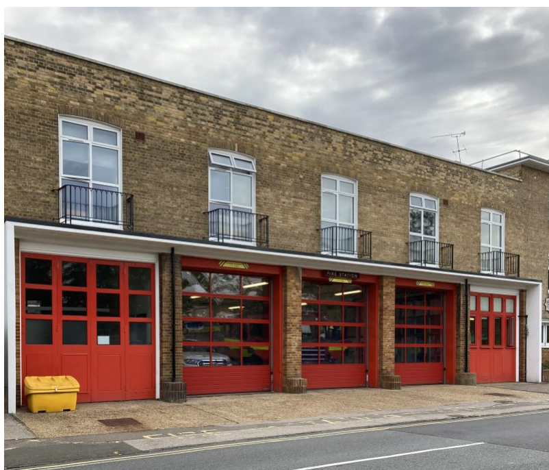
Epsom's Church Street Fire Station
