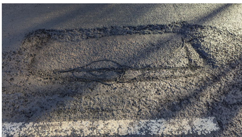
Cable exposed by pothole
