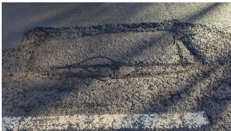
Cable exposed by pothole
