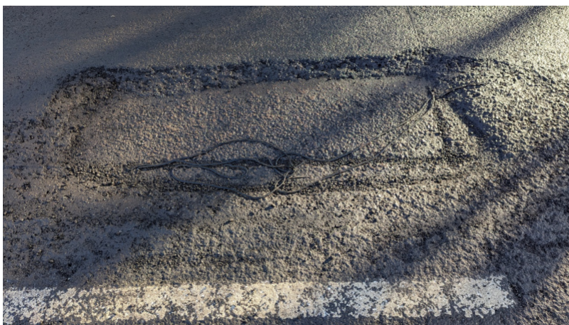
Cable exposed by pothole
