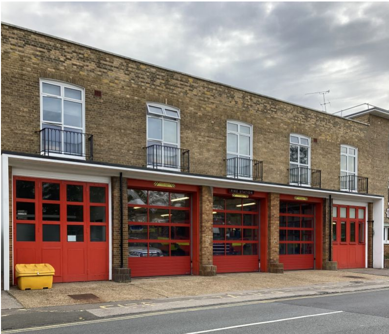
Epsom's Church Street Fire Station
