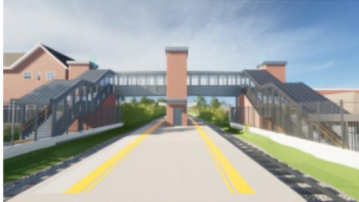
A new, covered footbridge will replace the existing structure at Stoneleigh station, providing full access via lifts or stairs to the central platform from both sides of the station. New lighting and security cameras will be installed on and around the lifts and bridge. The existing bridge structure will be removed, with the ticket office sited on the central island platform.
